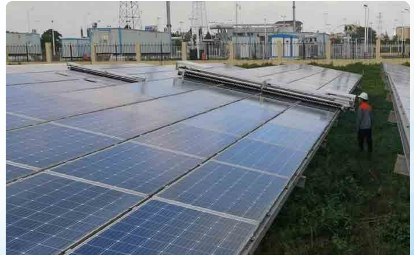
30 MW Solar Panels Cleaning Solutions in Hainan, China
