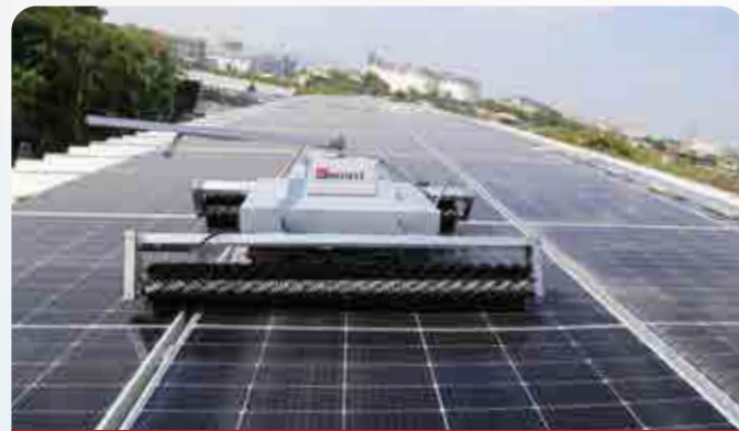
30.2KW roof of a cement plant
