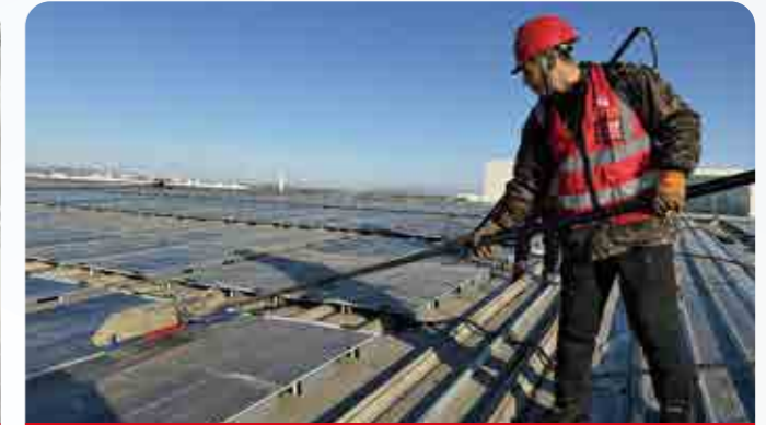
1.13MW in Beijing
