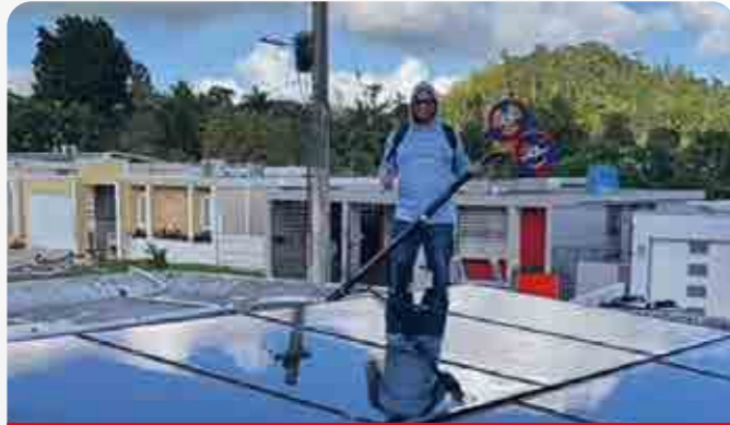
5KW Roof in the USA
